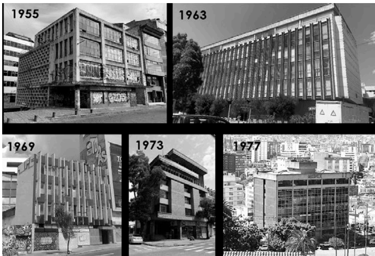
Figure 15. Mosaic of medium-sized office buildings various authors 1955 to 1980 in the city of Quito. Source: Photograph by the authors, June 2024
